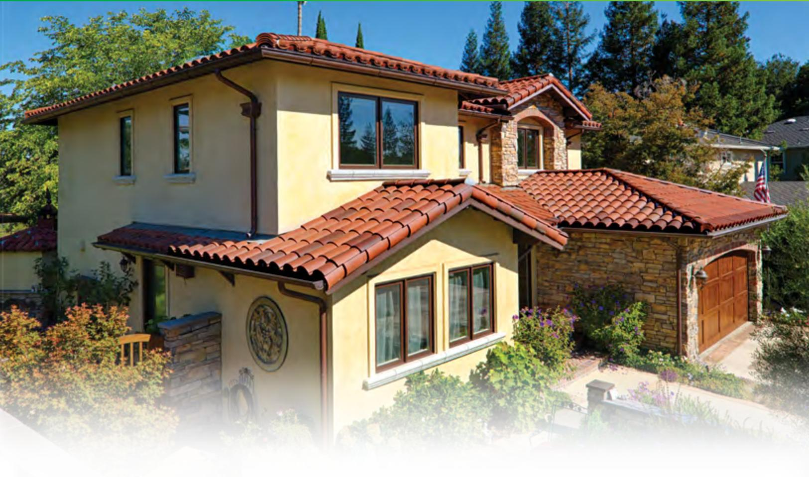
California Title 24, Part 6 Building Energy Efficiency Standards were established to reduce California's energy consumption. Cool roofs are important elements of an energy efficient structure, offering significant energy and cost savings. The California Energy Commission is updating the standards effective July 1, 2014, to include new prescriptive cool roof requirements in select zones for low-rise residential steep-slope roofs.
